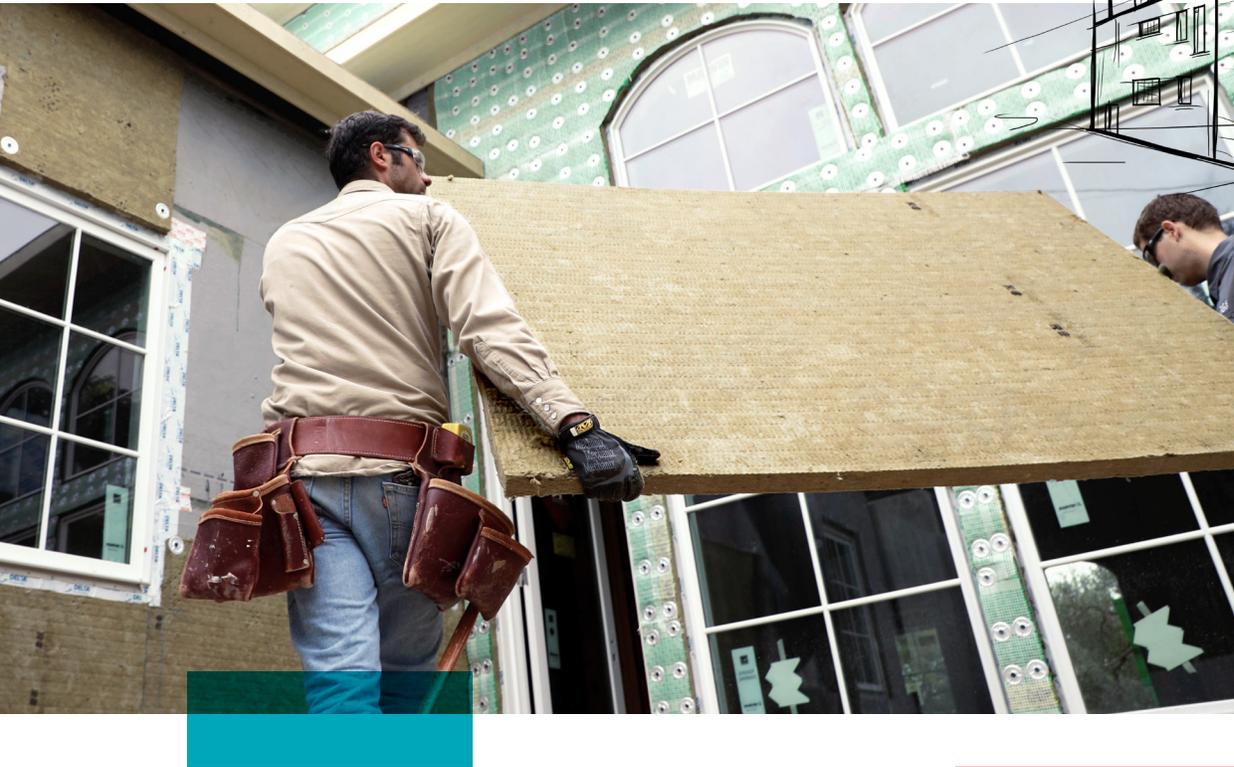
ROCKWOOL COMFORTBOARD™ 80 is a rigid stone wool continuous insulation board used as a non-structural sheathing product in residential construction.
